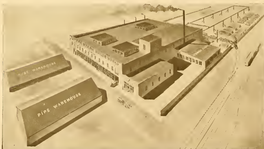
TOPEKA STEAM BOILER WORKS.
