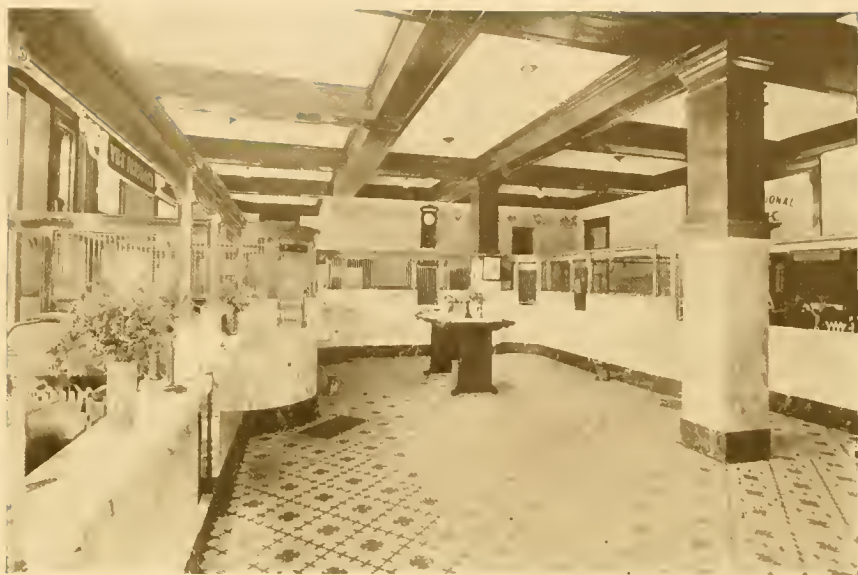
INTERIOR CENTRAL NATIONAL BANK.
