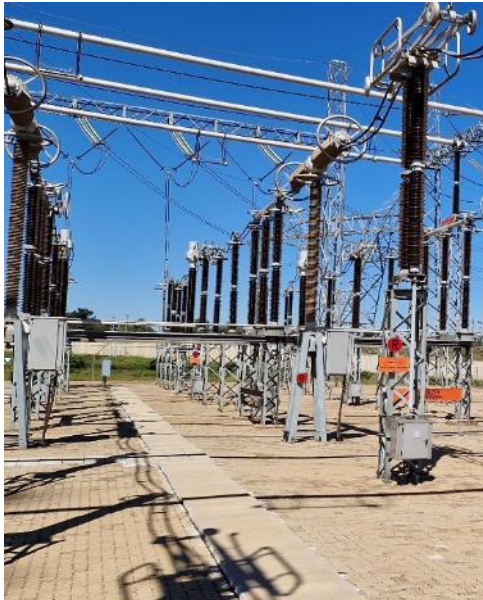
Figure 9-88: Cable duct in substation Thuso
