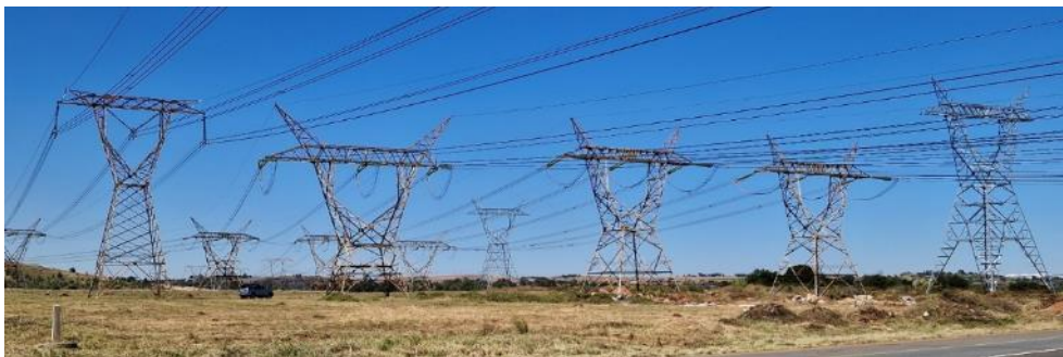
Figure 246: Inspected OHL section tower 1APO/THU013
