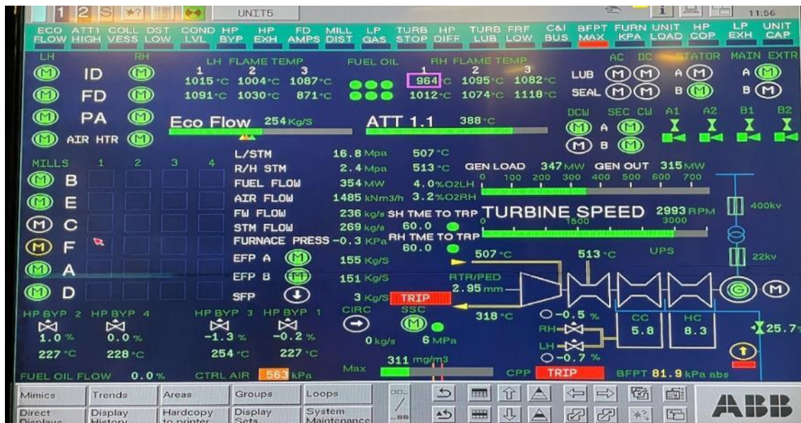
Figure 185: Boiler and steam conditions at Tutuka: air flow and fuel flow
