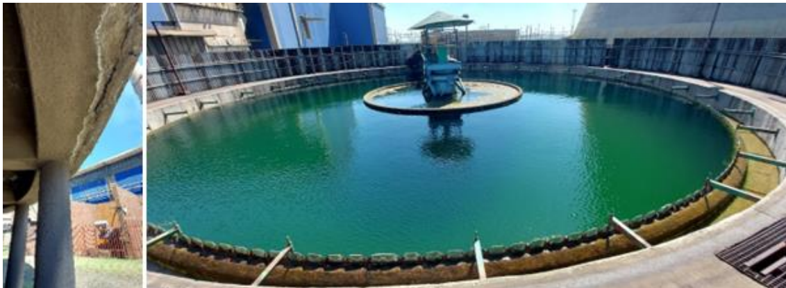
Figure 55: One of the clarifiers (right) and signs of wear and tear (left) at Camden
