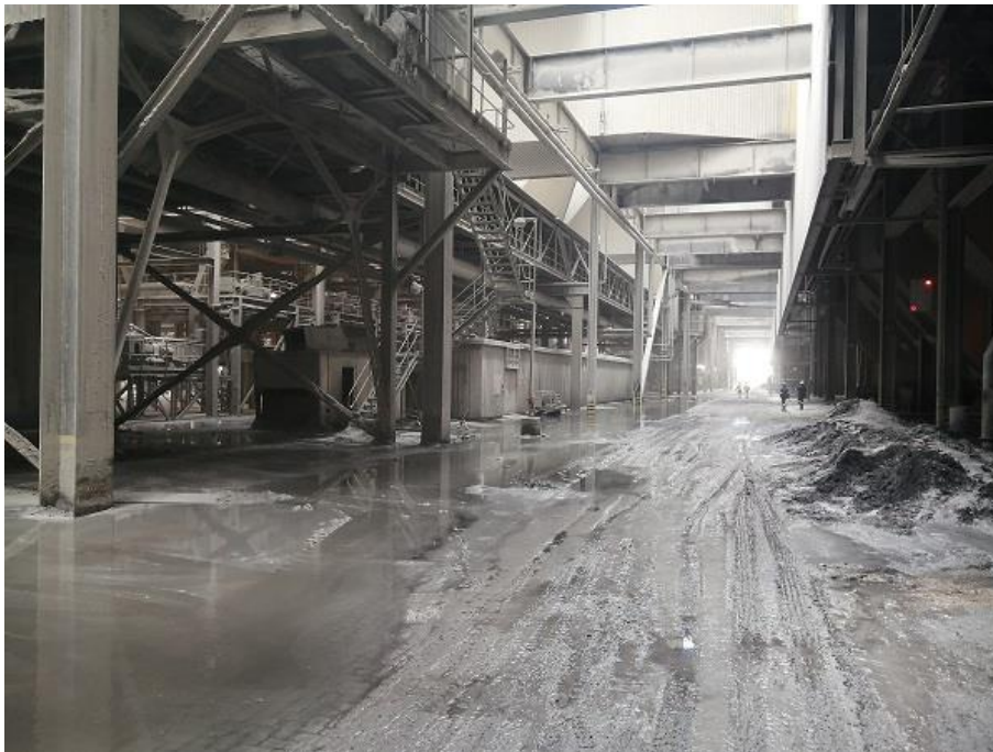
Figure 100: Ash in Kendal's boiler house
