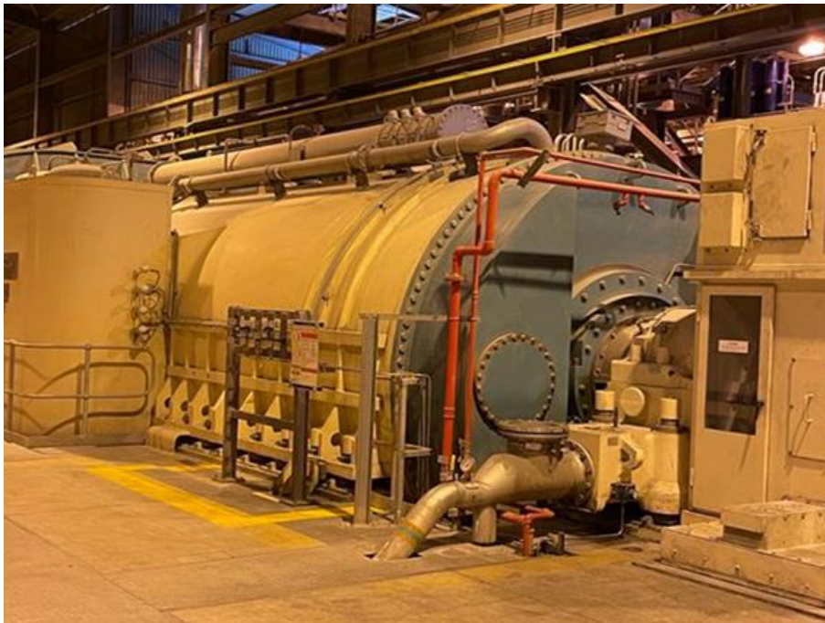
Figure 181: Good housekeeping at Medupi's turbine hall
