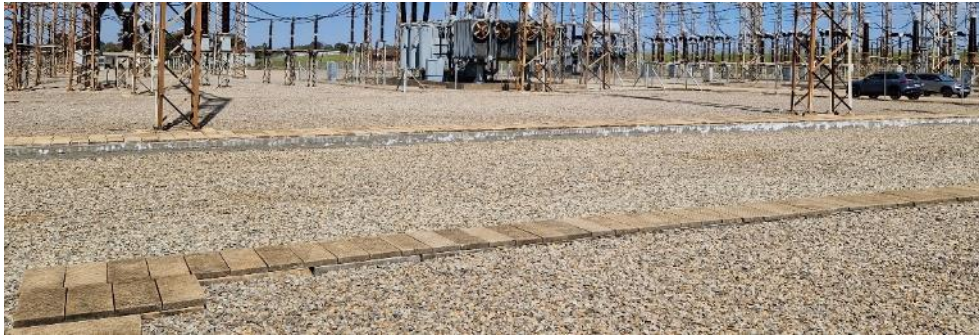
Figure 234: Example of cable duct substation Minerva
