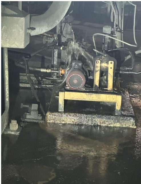
Figure 68: Water leakages in Grootvlei's dusty boiler house
