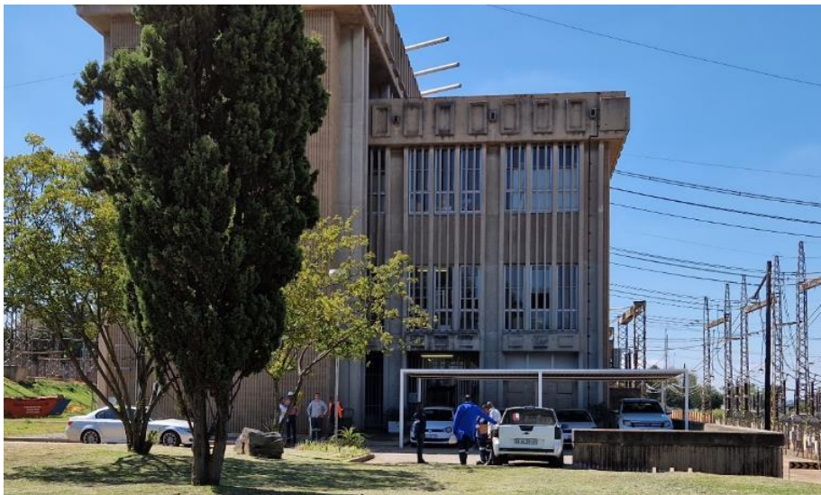
Figure 9-6: Operation Building substation Craighall
