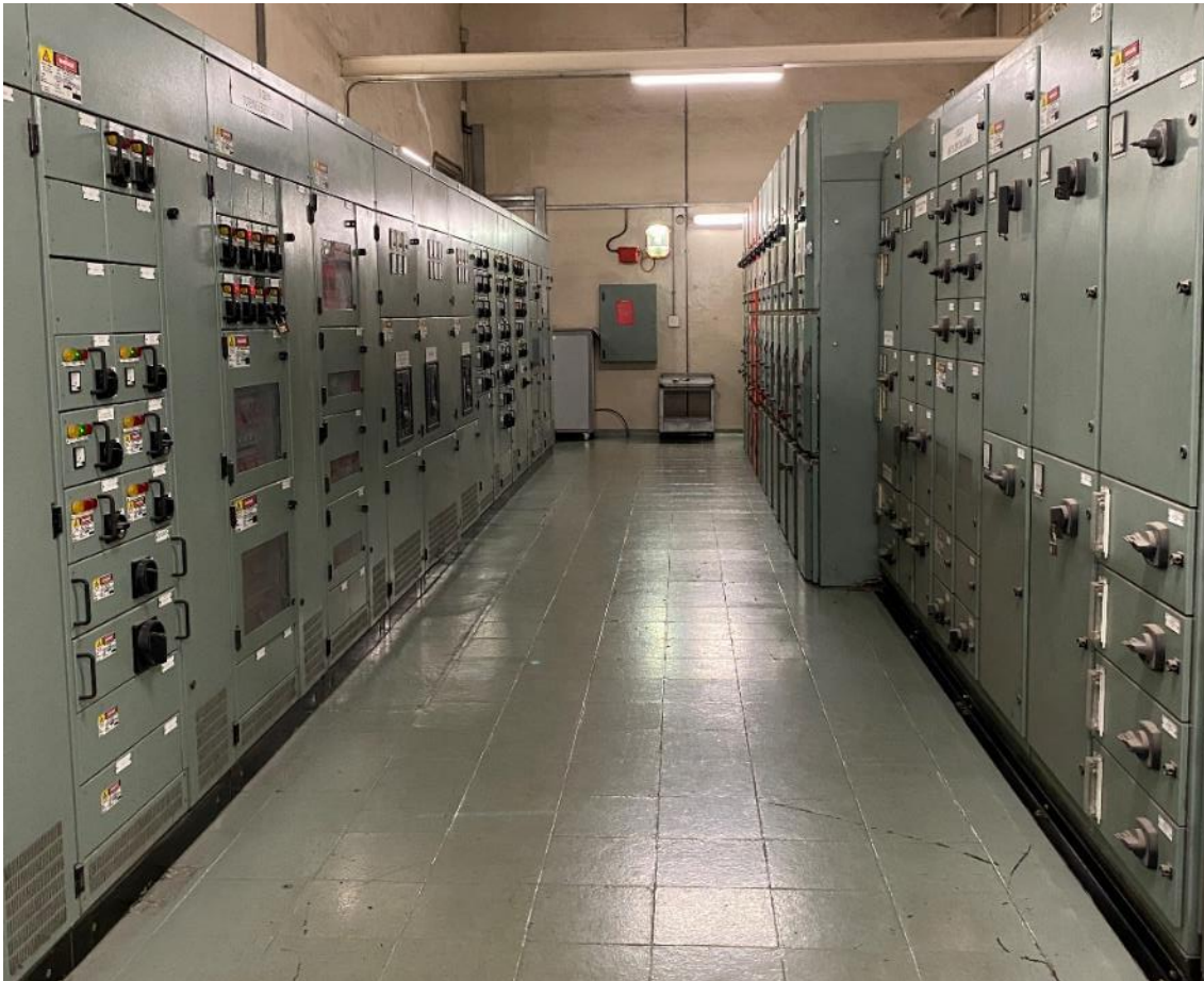
Figure 53: Clean and refurbished board rooms at Camden
