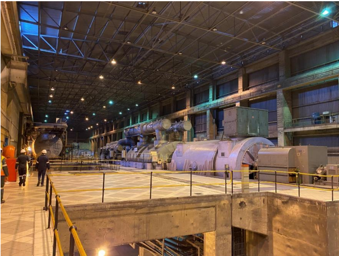
Figure 149: Reasonably clean turbine hall at Majuba power plant
