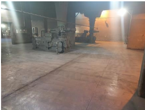
Figure 166: Matla's mill feeder floor at 16m level
