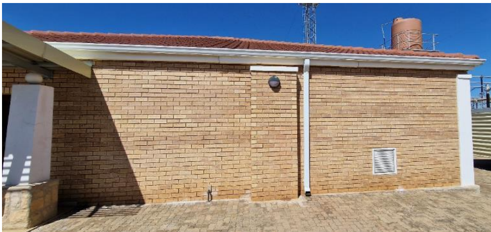
Figure 9-78: Operation Building of substation Thuso
