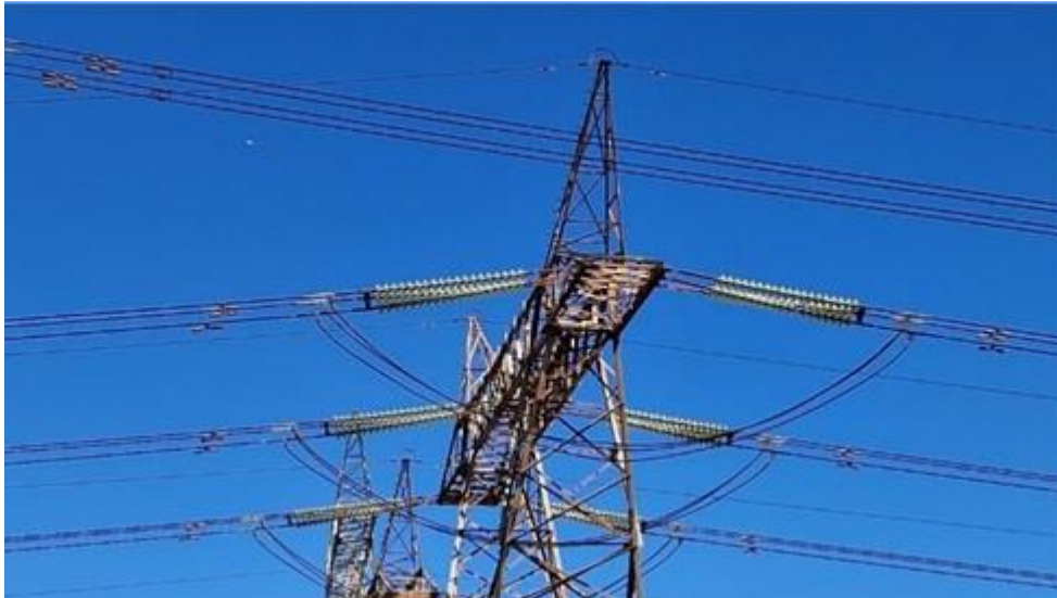
Figure 242: Insulation chains of 400 kV OHL
