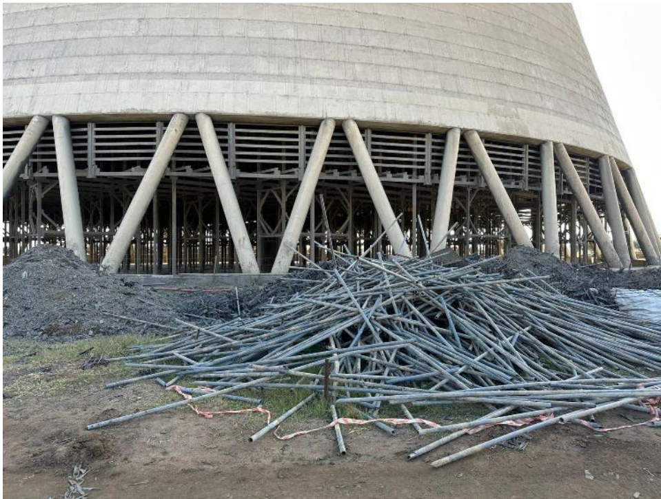
Figure 34: Removed filling of Arnot's cooling tower
