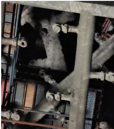
Figure 120: Choked spray nozzle at Kusile
