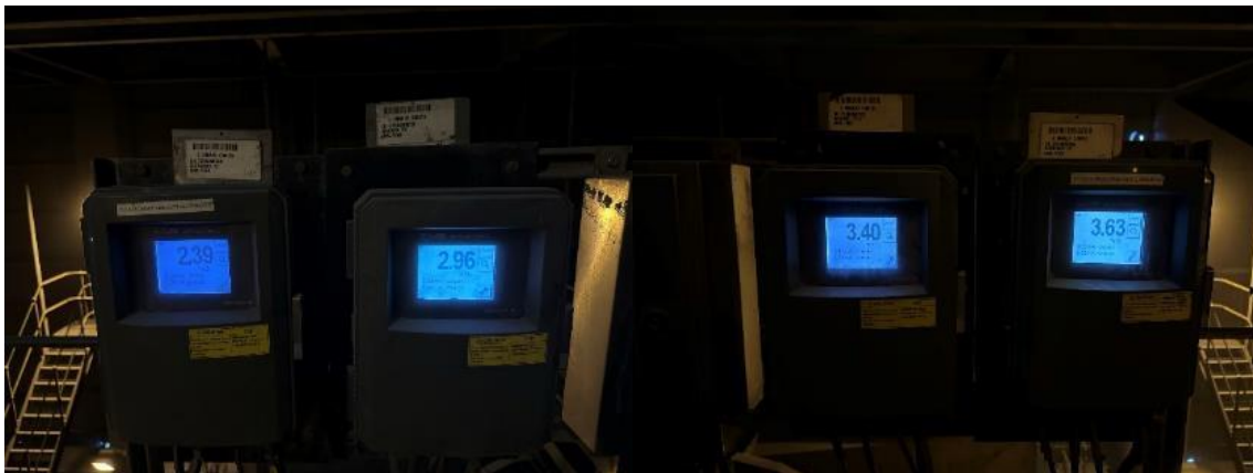
Figure 32: Measurement of oxygen in the flue gas at Arnot's Unit 3
