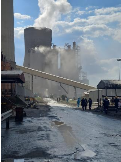
Figure 175: Dust pilot plant at Matla
