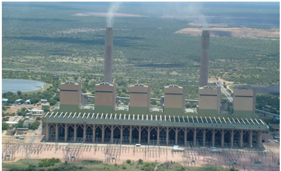
Matimba power plant, source: Eskom
