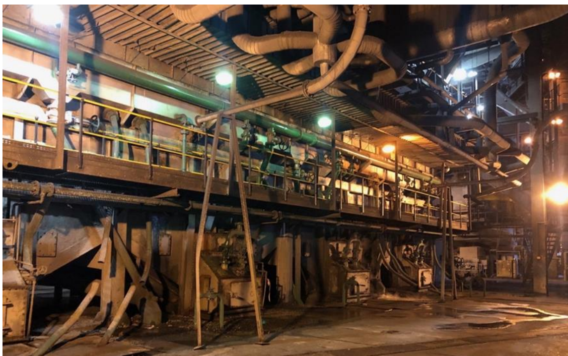
Figure 59: Duvha boiler level 0 m
