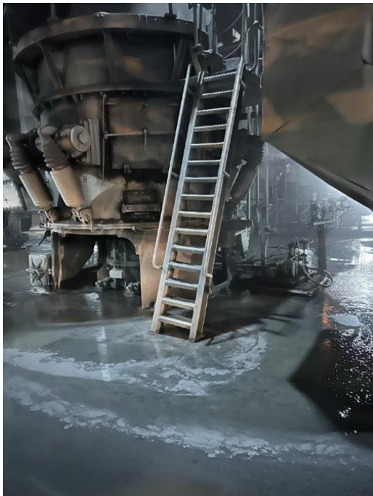
Figure 69: Flooded and wet floors at Grootvlei's 0 m level
