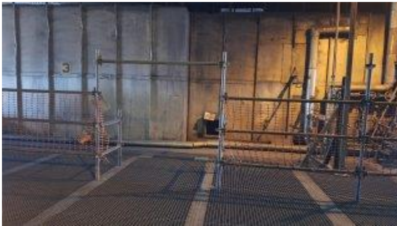
Figure 70: Fenced working area at Grootvlei boiler house
