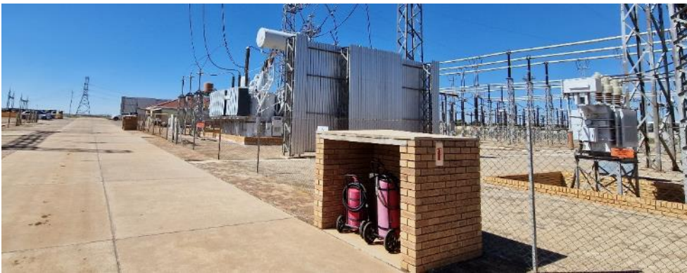
Figure 9-86: Transportation street and fence of substation Thuso
