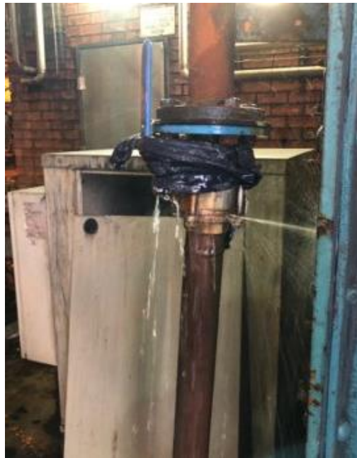
Figure 68: Water leakages in Grootvlei's dusty boiler house
