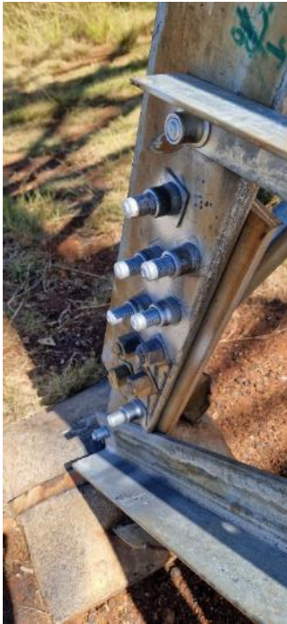
Figure 240: Self-locking nuts to avoid steel theft tower 1APO/THU013.
