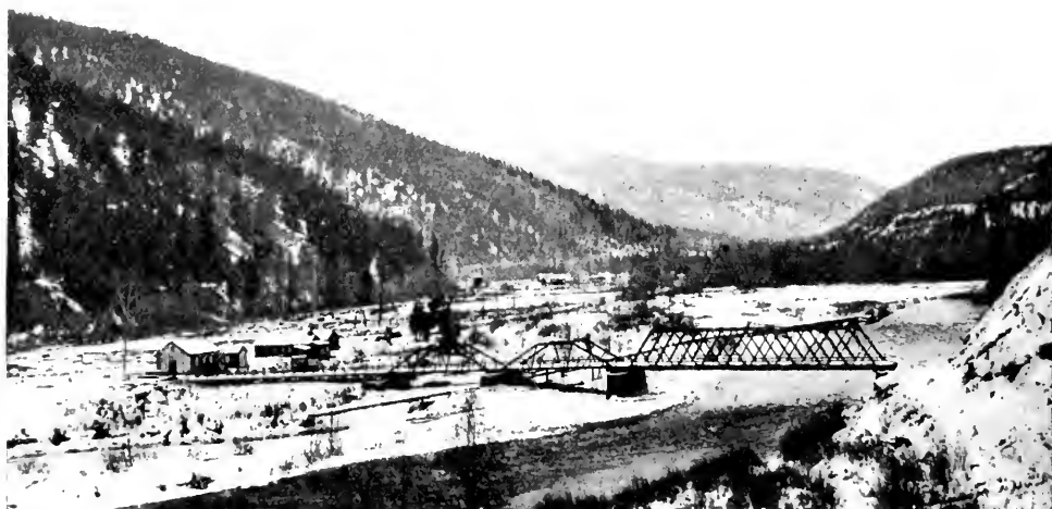
Tulameen river. Gauging station at highway bridge.
