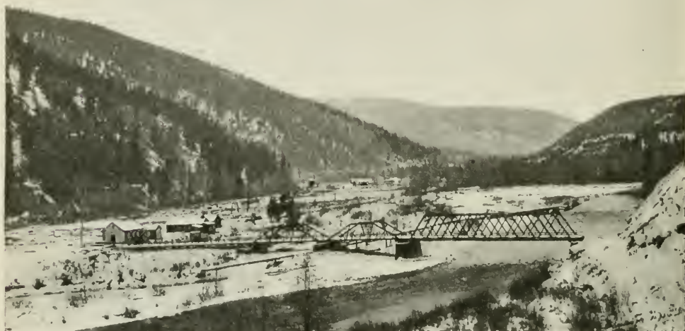
Tulameen river. Gauging station at highway bridge.
