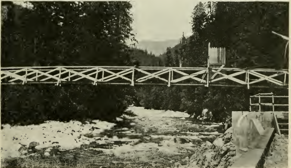
Showing intake of Vancouver Water Supply. Gauging section, Capilano creek, 10 feet above intake.
