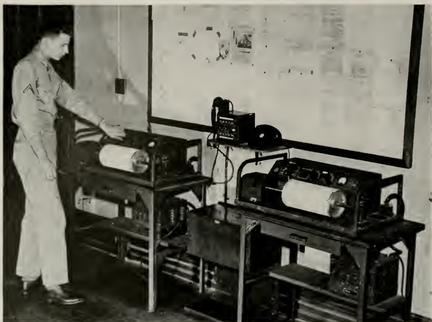
On the wire: A 12- by 18-inch reduction of the large working map goes on a facsimile "transceiver" for transmission over the Weather Map Network to all Air Force fields and bases in the country. The process takes about 20 minutes. The machine at the right is standby equipment
