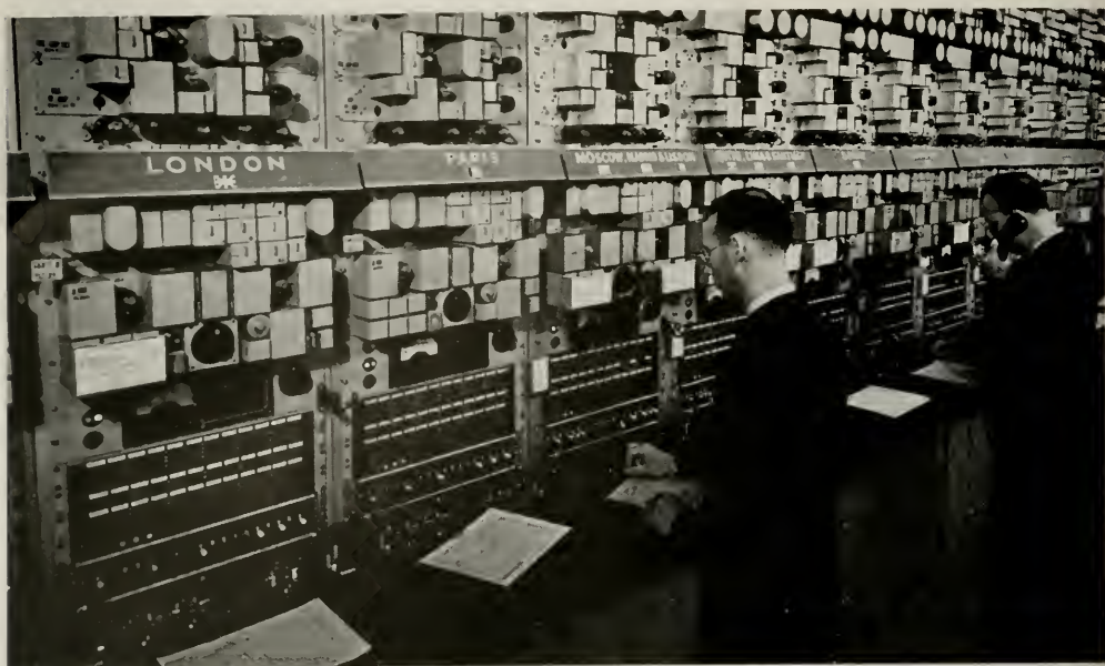
The overseas radio telephone circuit control room in the Long Lines building in New York
