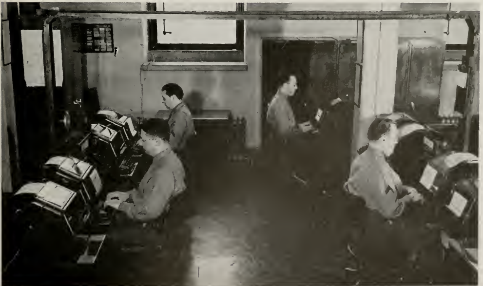
Teletypewriters at the headquarters of the New York State Police teletypewriter system, at Albany
