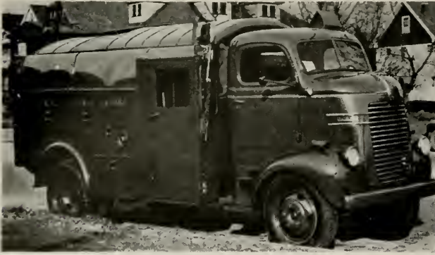
A Bell System construction truck with the newly designed crew compartment behind the cab
