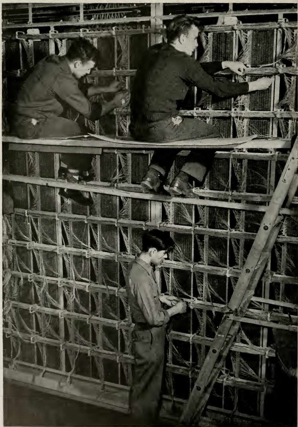
Installation of crossbar toll switching equipment in the Long Lines Department's headquarters building in New York—another step in the Bell System's operator toll dialing program. See the article beginning on the opposite page
