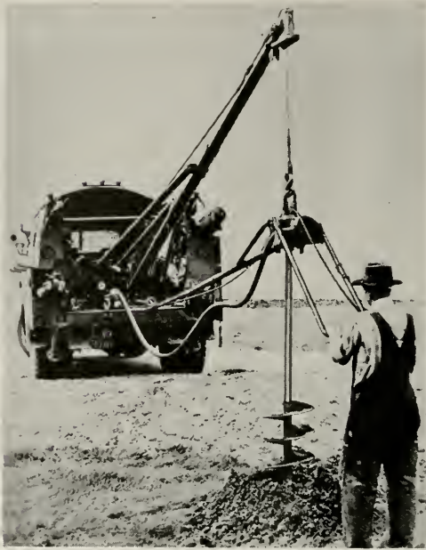
This light portable auger, suspended from the truck pole derrick and operated through a flexible shaft from its own small engine, is one of several types of earth-boring machines recently developed
