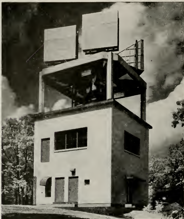
One of the seven intermediate hilltop stations along the route of the Bell System's new radio relay system between New York and Boston. Electro-magnetic lenses in the four horns atop the buildings receive and transmit long distance communications between the two cities. This is the station on Jackie Jones Mountain, near Haverstraw, N. Y.
