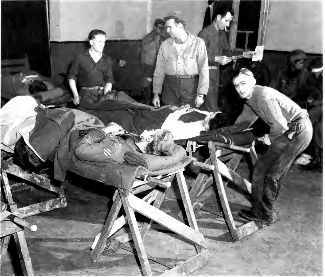
EVACUATION HOSPITAL RECEIVING WARD
