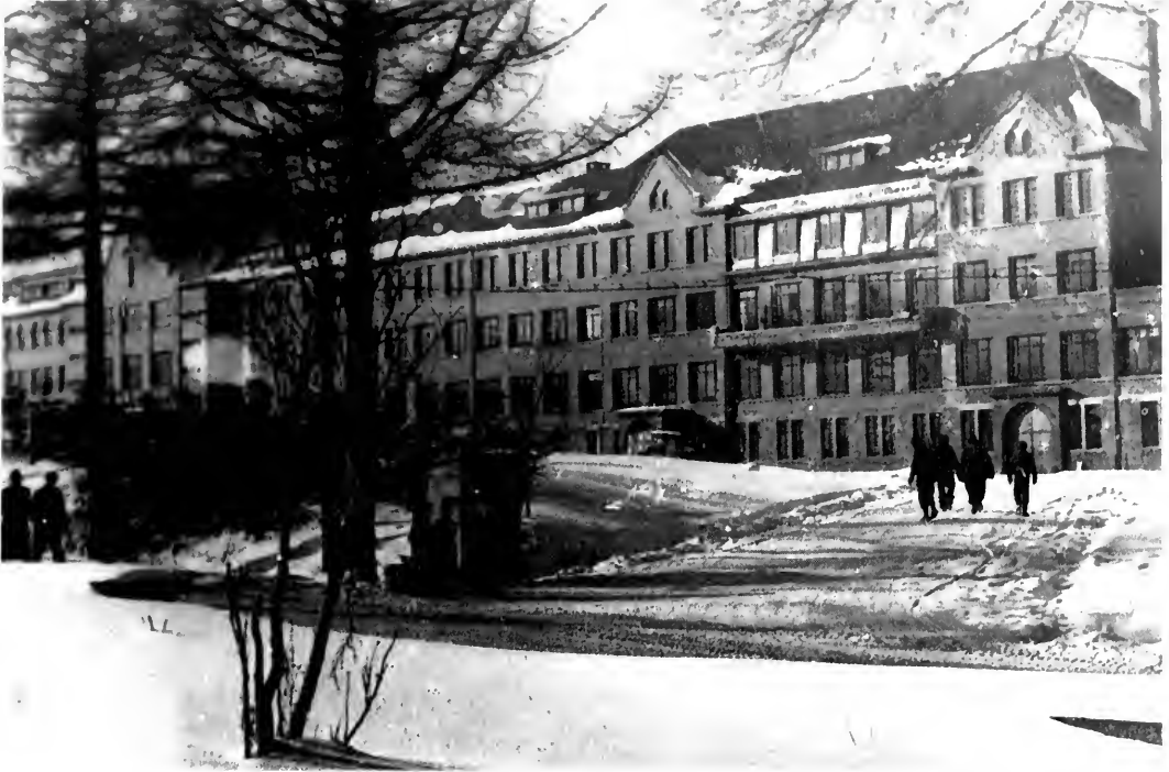
FORMER SCHOOL FACILITY HOUSING THE 130TH GENERAL HOSPITAL AT CINEY
