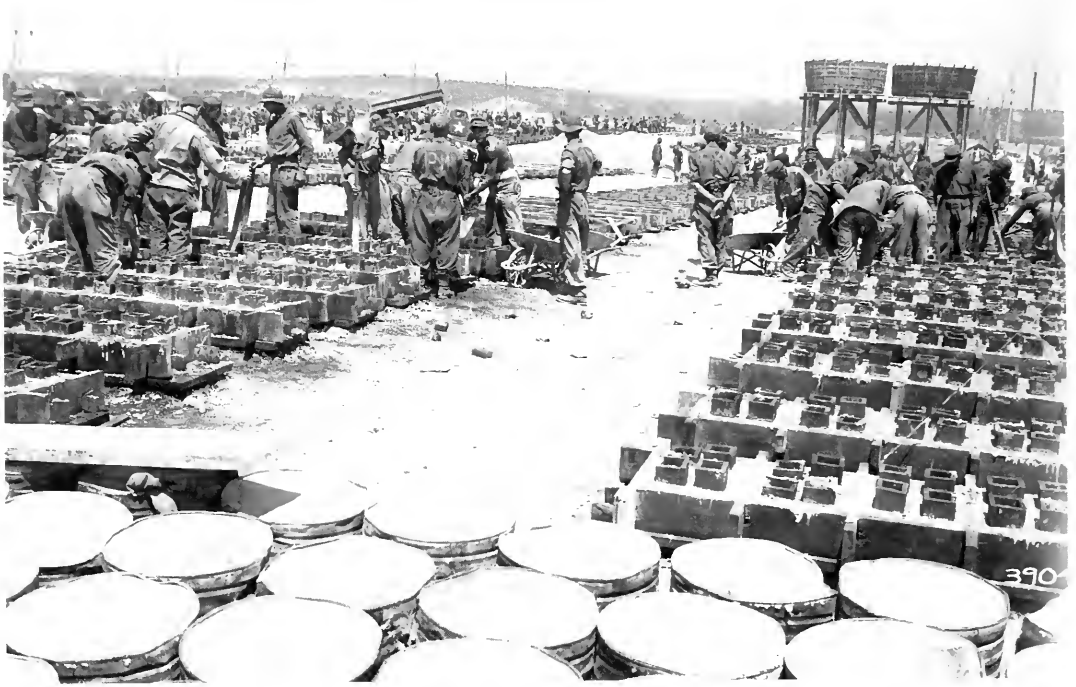
POW LABORERS AT DELTA BASE SECTION STAGING AREA near Marseilles
