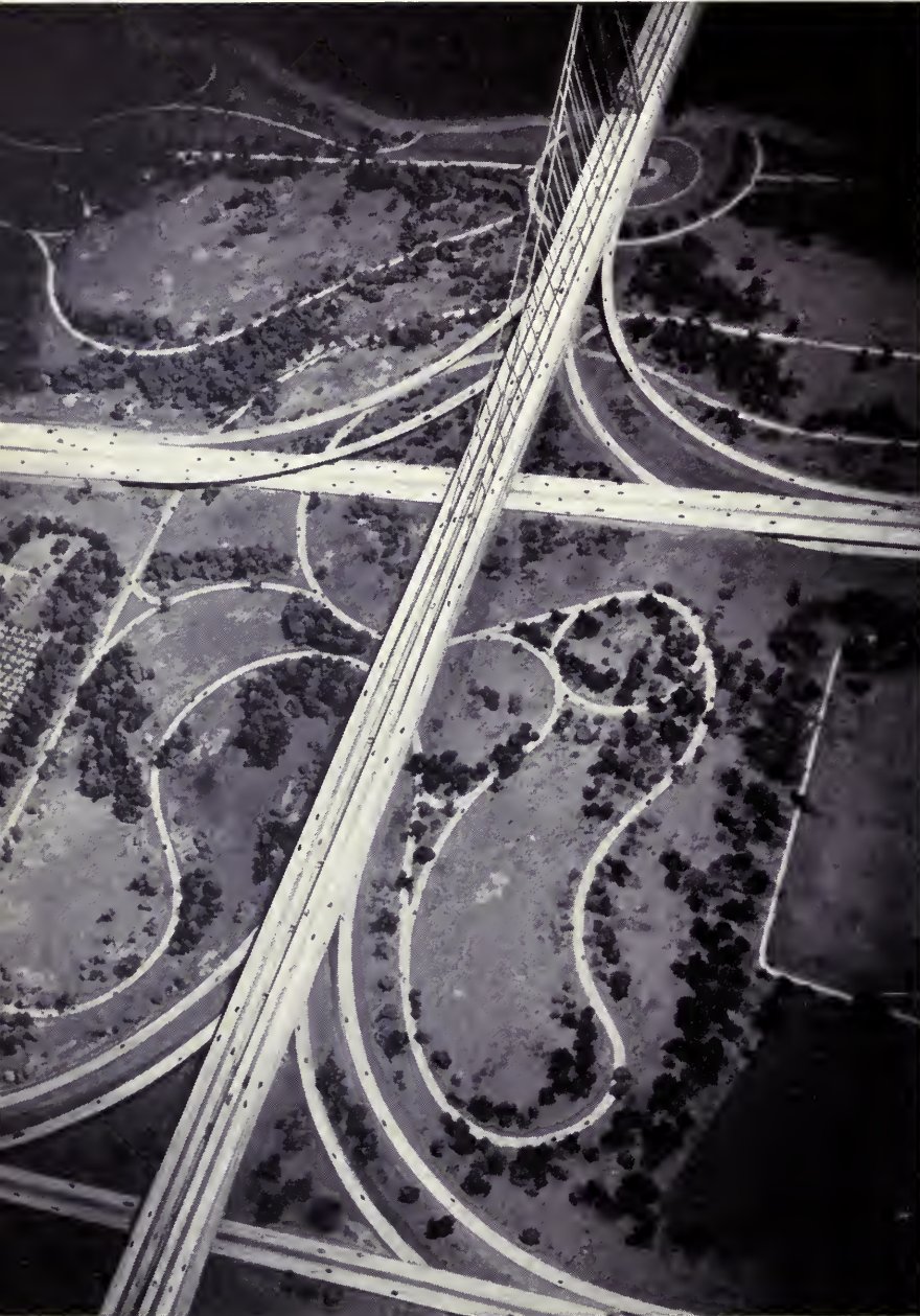
FUTURE BRIDGE PLAZA WILL ELIMINATE BOTTLENECK APPROACHES
