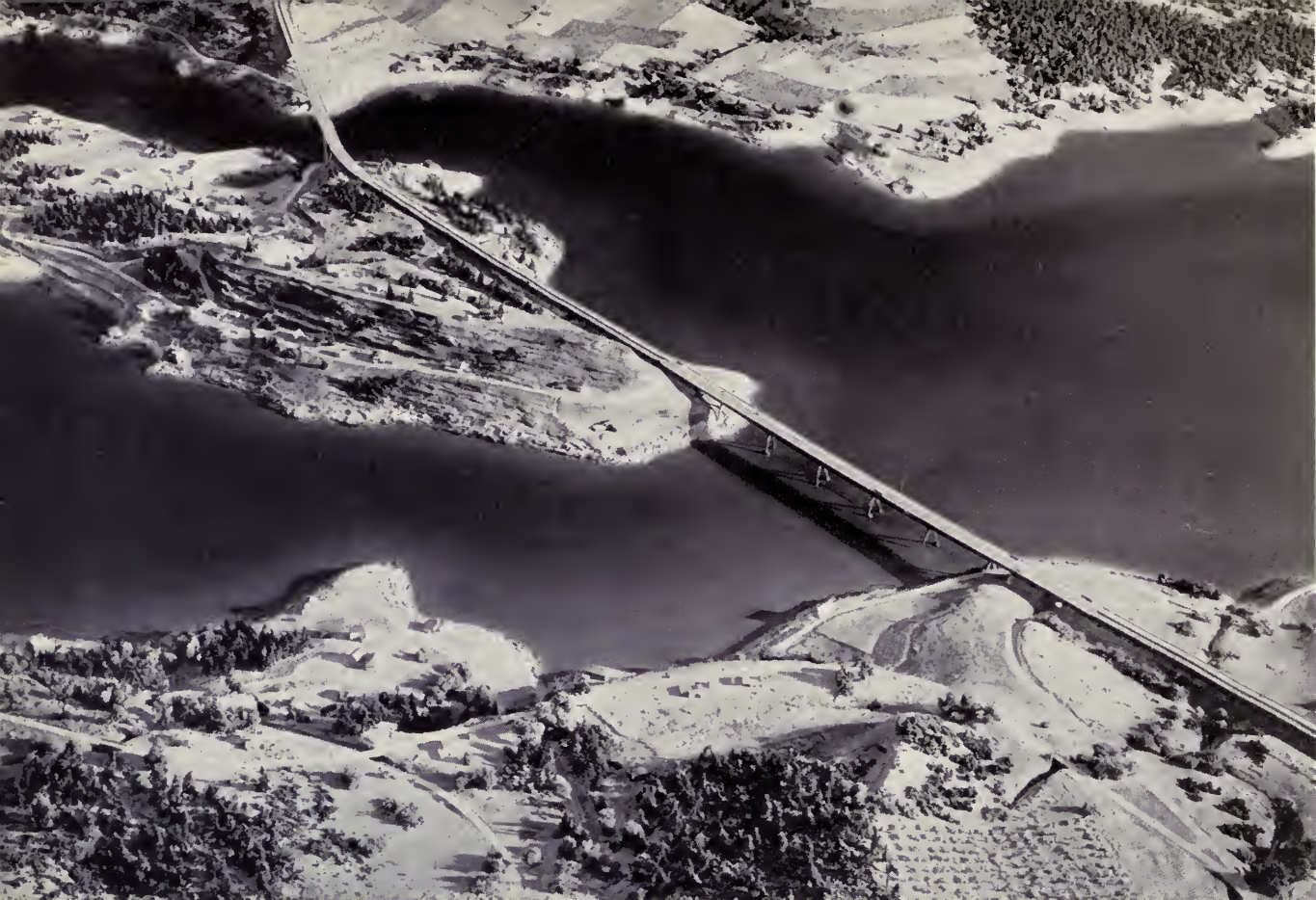
THE NATIONAL MOTORWAY CROSSES A LARGE LAKE
